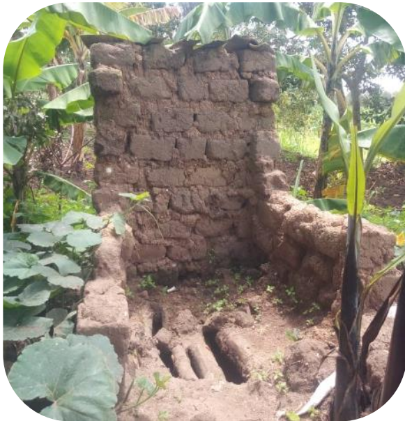
Mukarubayiza Melanie's latrine wasn't properly constructed.
