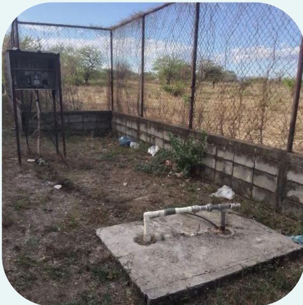
Contamination from the septic tank seeped through the ground until it reached the prison's water source.
