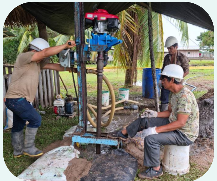
Living Water staff drill a new borehole until they reach a safe water aquifer 60 meters underground.
