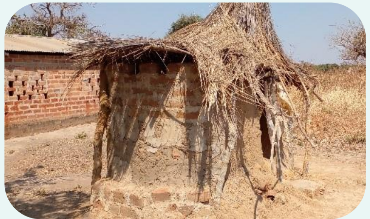
The church congregation tried to construct a latrine at the church, but the hole is too shallow, and the roof is caving in.
