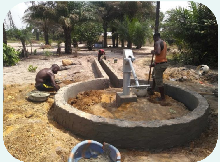
The construction crew works to lay a concrete base for a new hand pump.
