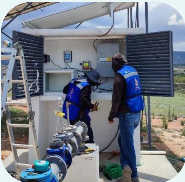
The construction crew works on installing a new chlorination center for the community's piped water system.
