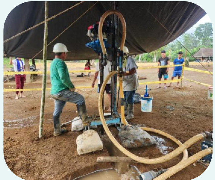
Living Water staff use a drill rig to drill 18 meters to access a safe water aquifer. This aquifer will serve as a reliable source of safe drinking water after being chlorinated and sealed from contamination.
