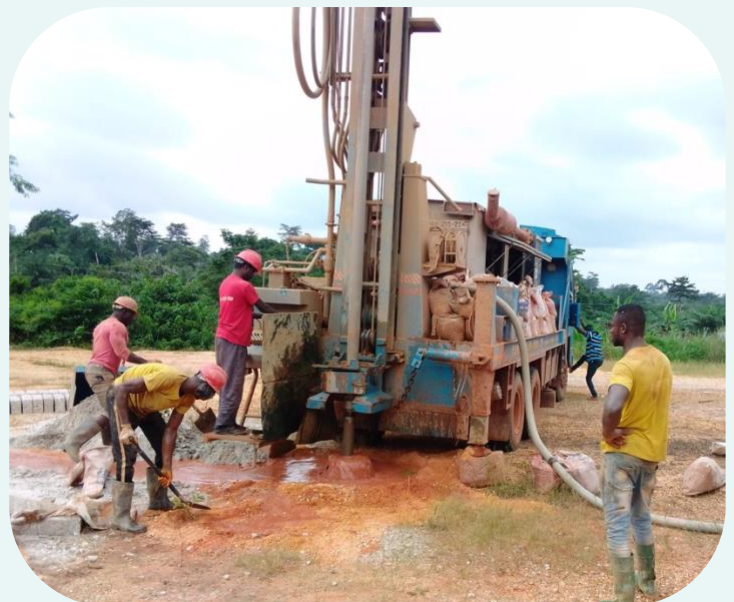
Construction is underway! The Living Water staff work to drill a borehole until reaching a safe water aquifer.
