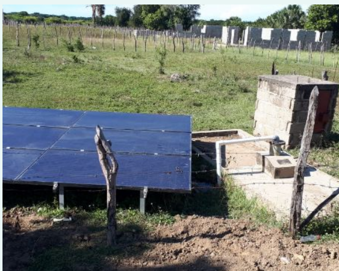
The new piped water source is powered by solar panels, ensuring that community members have access to water regardless of access to electricity.
