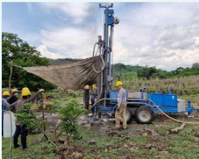
The Living Water team drilled 77 meters to access an underground aquifer. After testing the water to ensure it was safe, the staff treated the borehole with shock chlorination.
