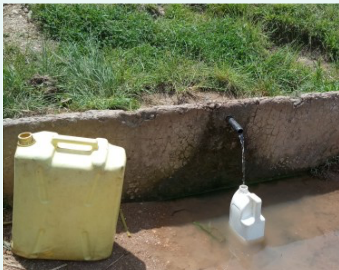
This unprotected spring is exposed to contaminants, and its supply is scarce during the dry season, making this source unsafe and inconsistent.
