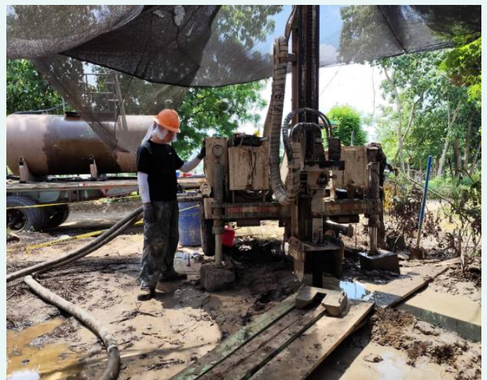
The Living Water staff drills 56 meters to reach a safe, underground aquifer. After treating and testing the water for safety, they will manually install PVC piping and a new hand pump for easy access.
