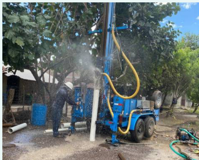
The Living Water staff drills 24 meters to reach a safe, underground aquifer. After treating and testing the water for safety, they will manually install PVC piping and a new hand pump for easy access.
