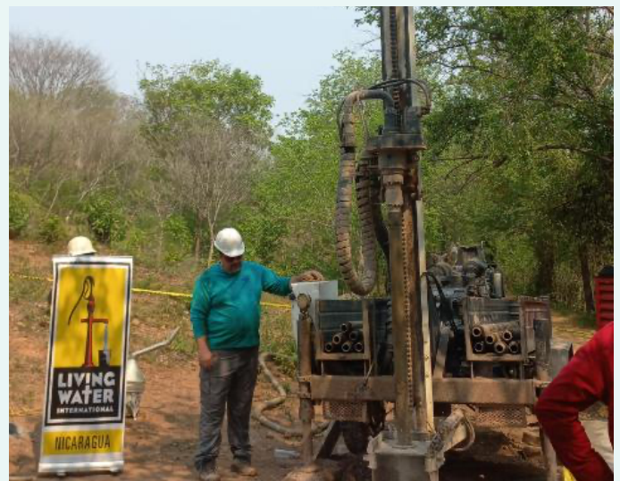
The Living Water staff drills 61 meters to reach a safe, underground aquifer. After treating and testing the water for safety, they will manually install PVC piping and a new hand pump.
