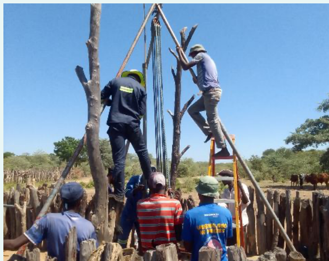
The Living Water staff drills 50 meters to reach a safe, underground aquifer. After treating and testing the water for safety, they manually install PVC piping and a new hand pump.
