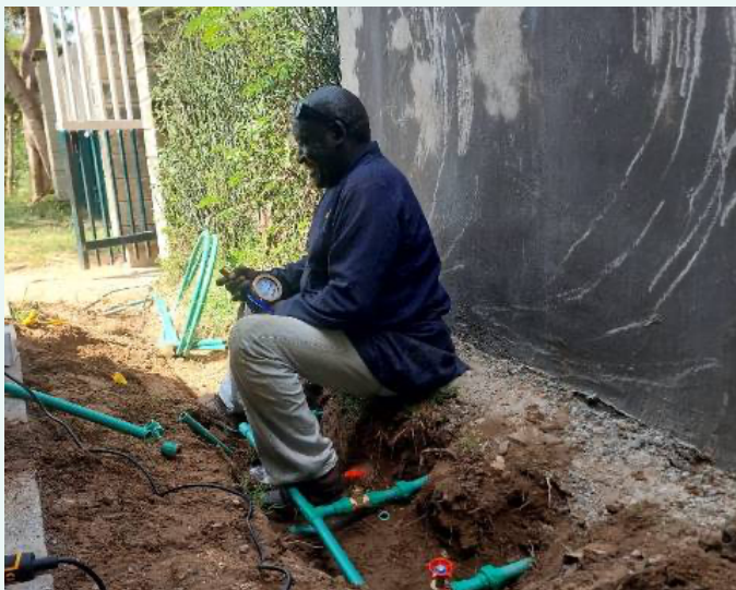
After drilling until reaching a safe underground aquifer, Living Water staff tests the water's safety and installs over 1,000 meters of PVC piping and a solar submersible pump. Finally, they will build a stand with three taps.
