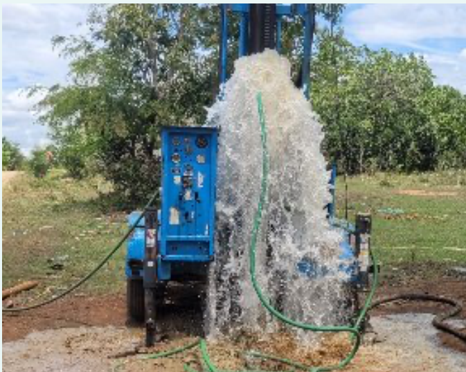
The Living Water staff drills 40 meters to reach a safe, underground aquifer, allowing the borehole to express itself. After treating and testing the water for safety, they will install PVC piping and a new hand pump.
