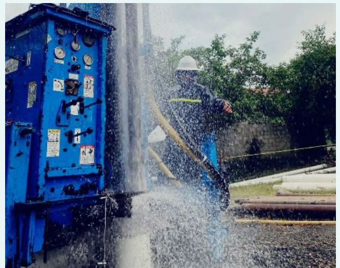
Living Water staff drilled 54 meters to reach a safe, underground aquifer and installed PVC piping and a new hand pump.
