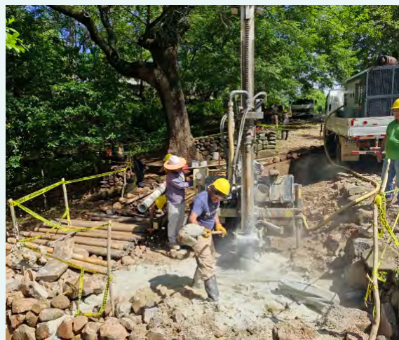
Living Water staff bring safe water to La Picota, reaching an aquifer at 50 meters below ground.
