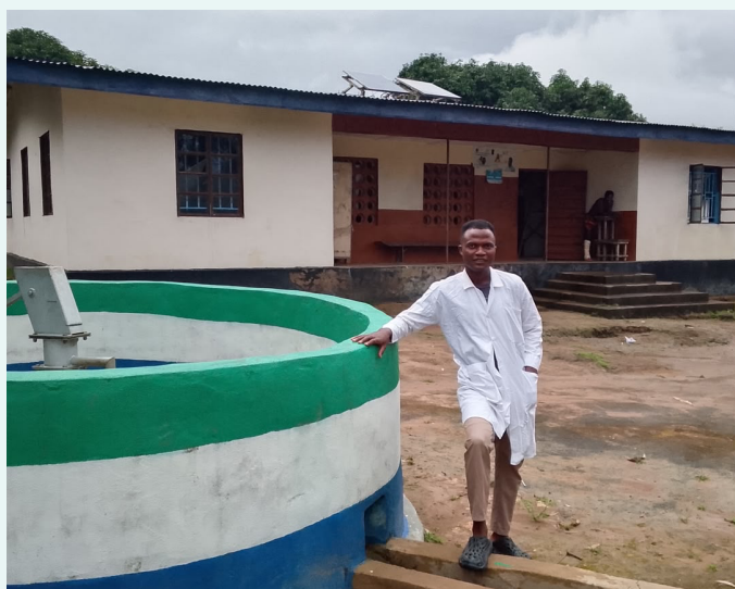
Eddie stands next to the new water source, grateful to have easy access to safe water throughout the workday.
