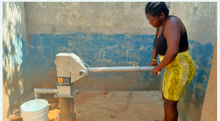
Residents are thankful to have a restored hand pump, ensuring safe water near their homes.
