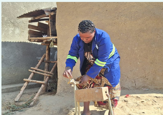
With the plumbing skills Kasande learned from Living Water staff, she works on repairing some pipes.
